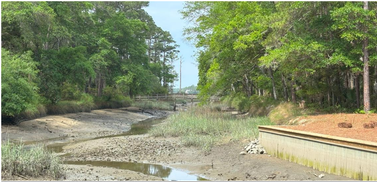
Figure 4. Multi-phase installation of Envirolok on Kiawah Island. Note difference in vegetative cover at different phases.
